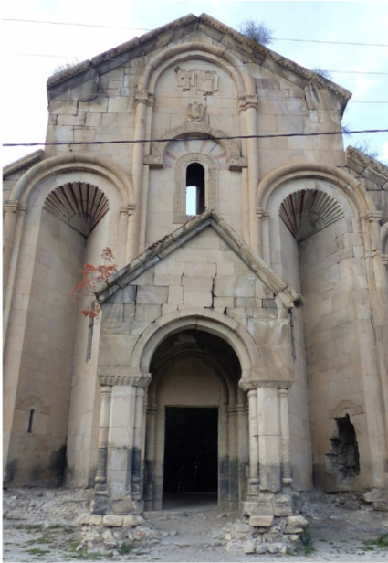
Fig. 3. Oshki's South Porch
