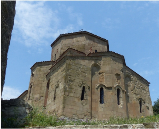
Fig. 2. Jvari from the East-south
