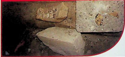
„Innovative“ methods for restoration-conservation...
